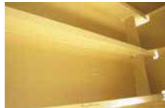
Water ballast tank coatings
