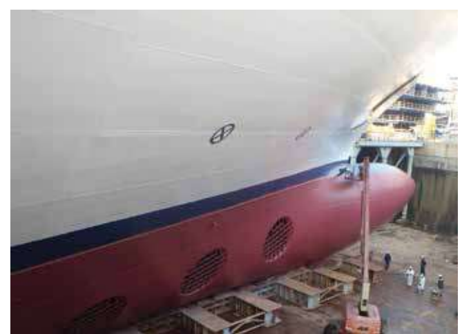
Antifouling coating now being applied (large vessels)
